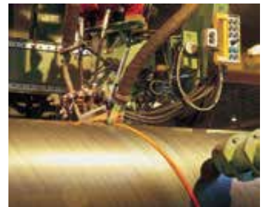
Internal & external welding
